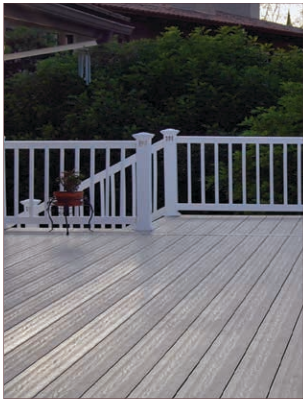
SLATE GREY DECK & VINYL RAILING
